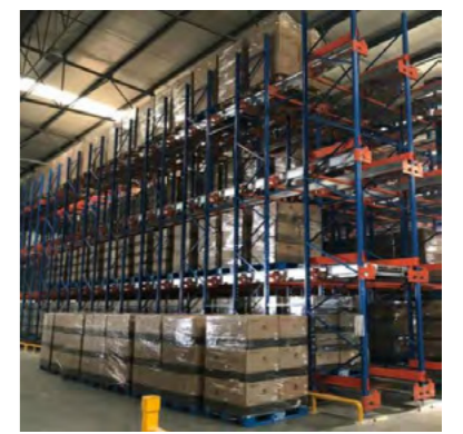
Shuttle Channel Pallet Racking
