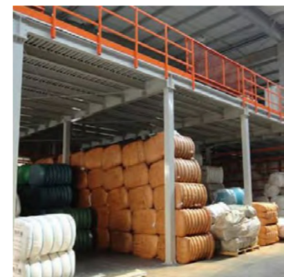
Multi- Level Platform Steel Structure
