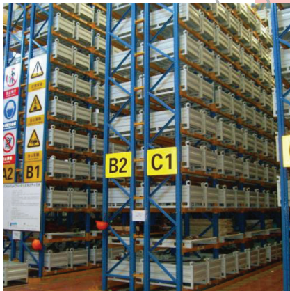
High Density VNA Storage Pallet Racking
